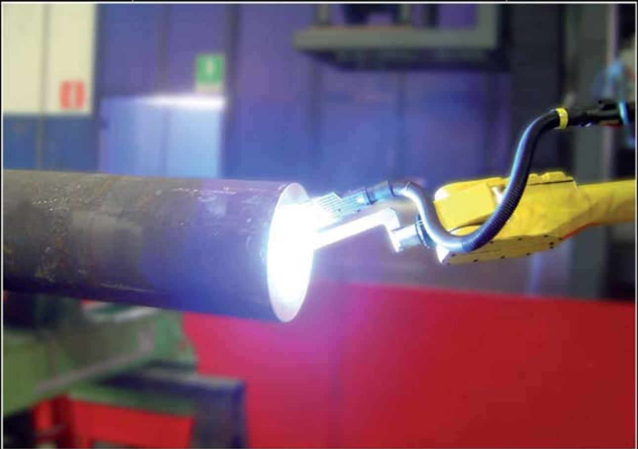
CLADDING OF PIPE
