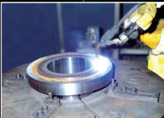
CLADDING OF FLANGES
