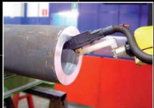
CLADDING OF PIPE
